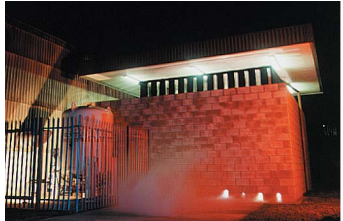
Cryogenic Test Facility/Explosion Proof Chamber.
